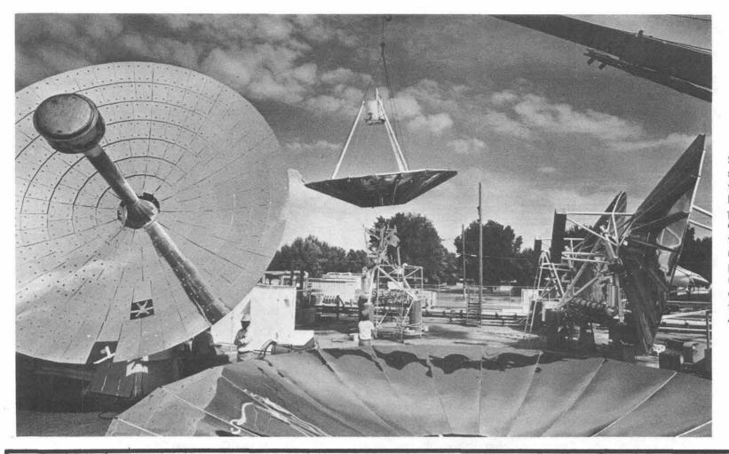
SOLAR REFLECTORS, possible prototypes of a system to power a fashion knitwear manufacturing plant near Shenandoah, Ga., are moved into position in the solar test area near Bldg. 832. Components of the system are undergoing test and evaluation by Small Power Systems Application Division 4725 under Jim Leonard.
